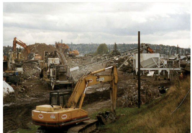
RW Rhine Demolition
