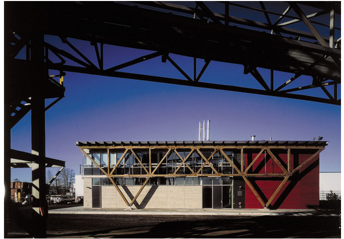
City of Vancouver Materials Testing Laboratory Busby + Associates
