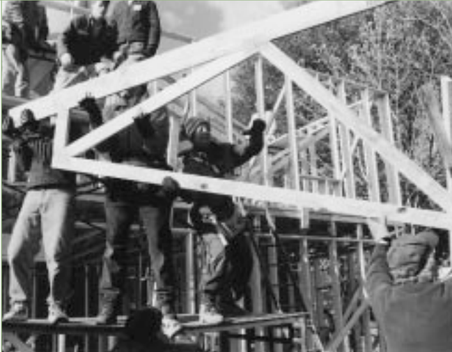
RAISE HIGH THE ROOF TRUSSES
