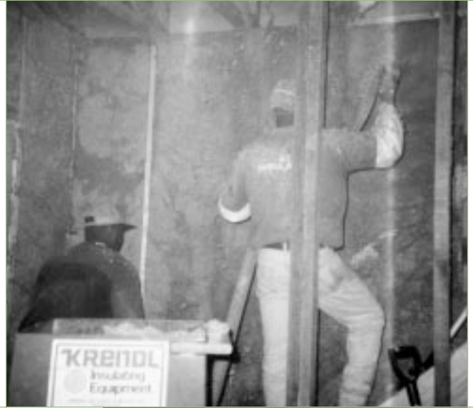
INSTALLING WET-BLOWN CELLULOSE INSULATION
