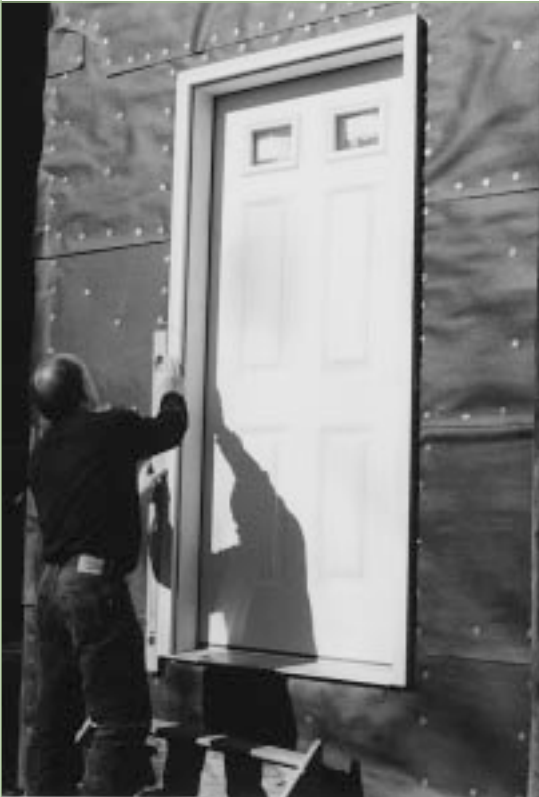
EXTERIOR DOOR INSTALLED
