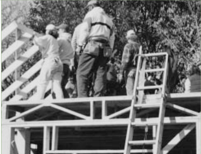
OPEN-WEB FLOOR TRUSS
