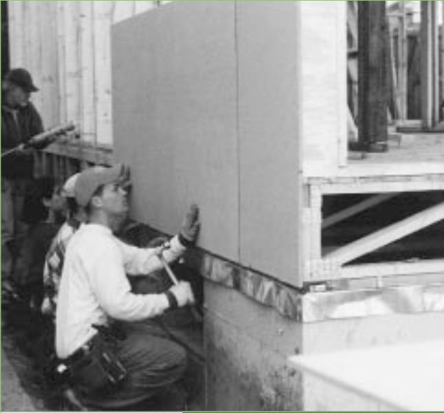
INSTALLING HOMASOTE SHEATHING
